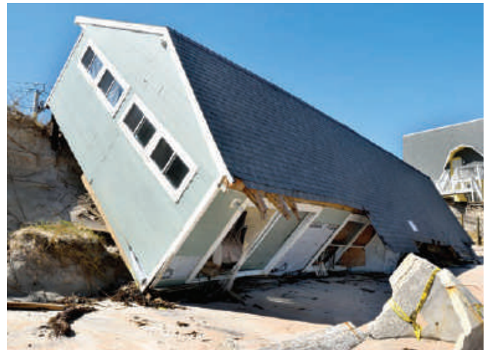
Damage by Hurricane Irma.
