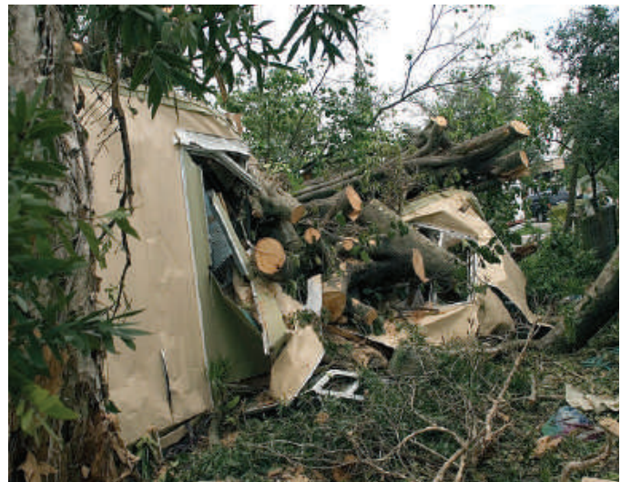
Hurricane damage to mobile home in Davie, FL.
